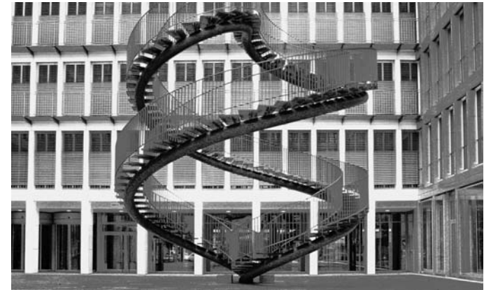
ILLUS. S1-11 KPMS Building, courtyard stair, Munich, Germany
