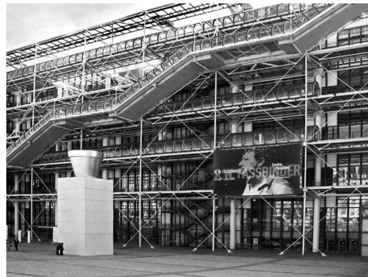
ILLUS. S1-14 Pompidou Center, Paris—exterior escalator—(Renzo Piano, architect)
