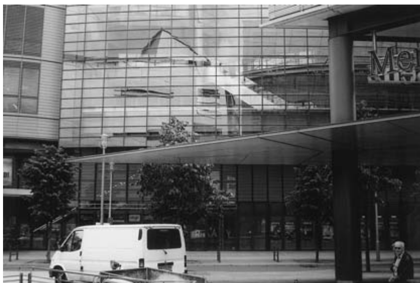
Fig. 23.1 Building with cantilevered canopy, Berlin.
