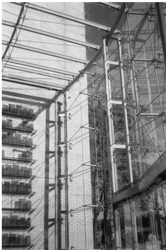
Fig. 24.5 Atrium, Learning Centre, Leeds Metropolitan University.
