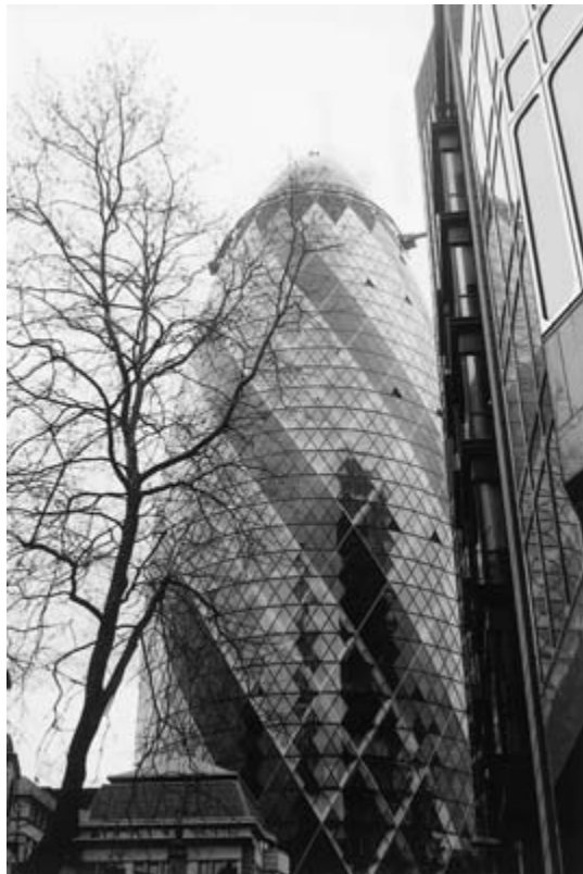
Fig. 14.2 Swiss Re building, London.
