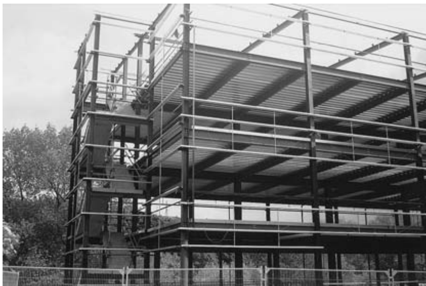
Fig. 22.1 Steel-framed office building under construction.
