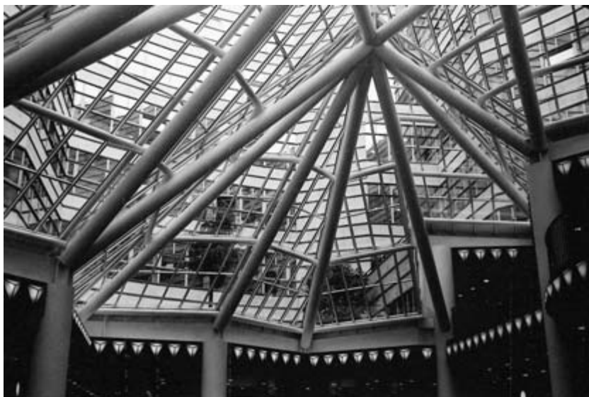
Fig. 1.2 Roof structure of Quartier 206 shopping mall, Berlin.
