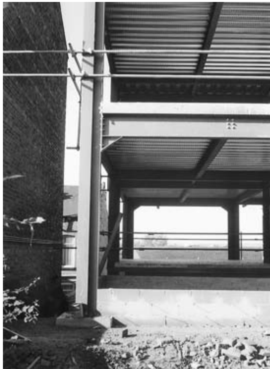
Fig. 9.2 Steel-framed building under construction.
