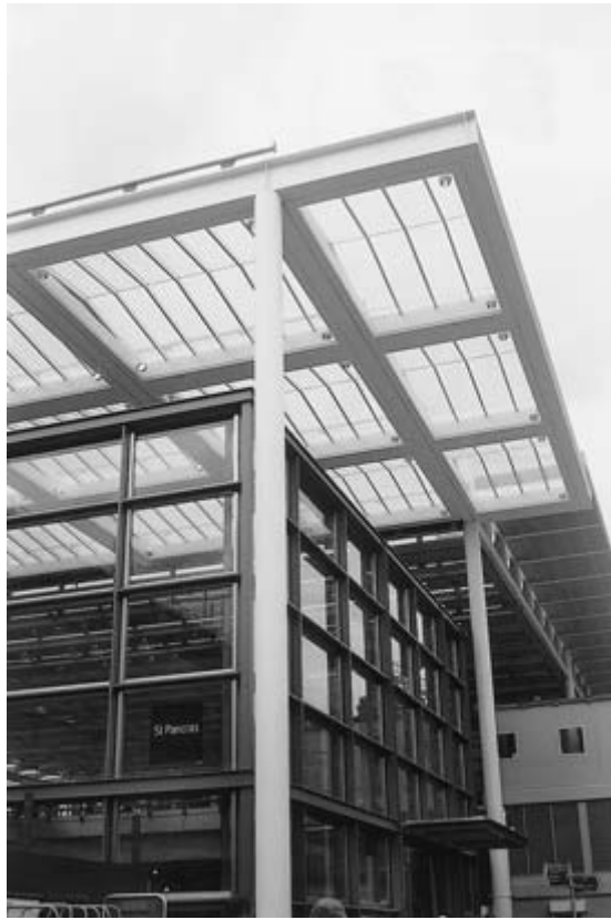
Fig. 10.8 St Pancras 'interim' railway station, London.
