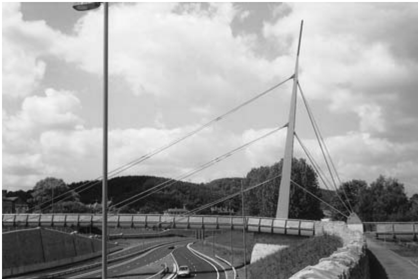
Fig. 17.3 Cable-stayed bridge, Bingley bypass, West Yorkshire.
