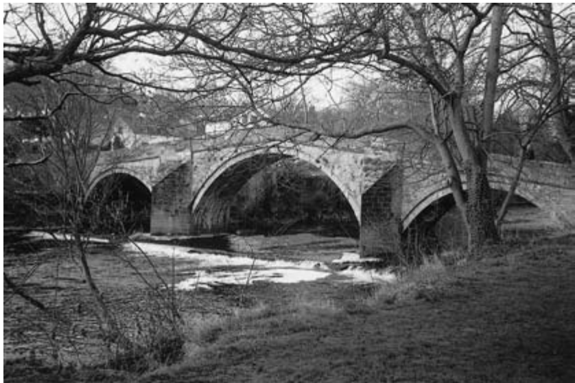
Fig. 21.1 Stone arch bridge.
