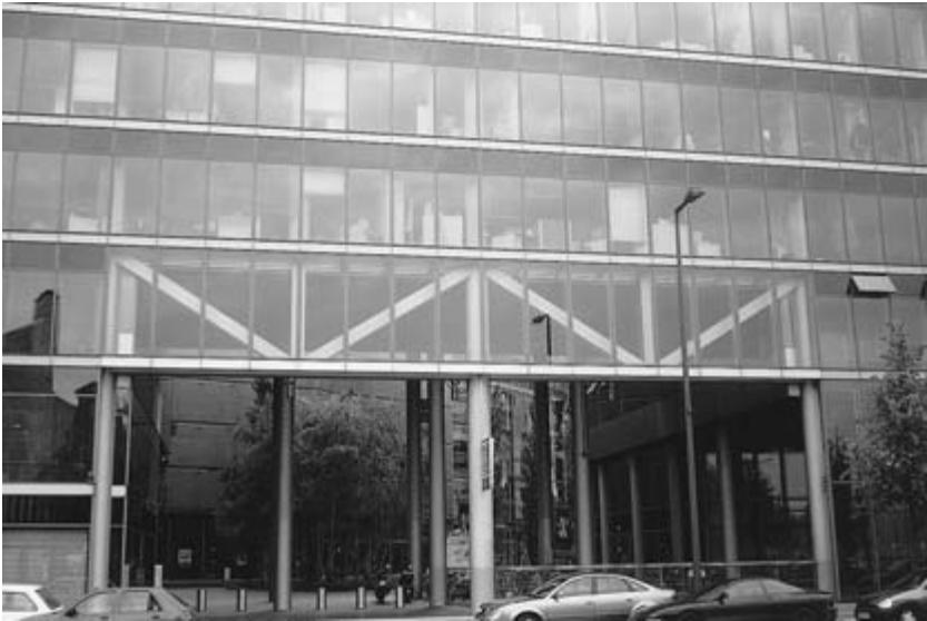
Fig. 12.5 Truss in façade, Sony Centre, Berlin.
