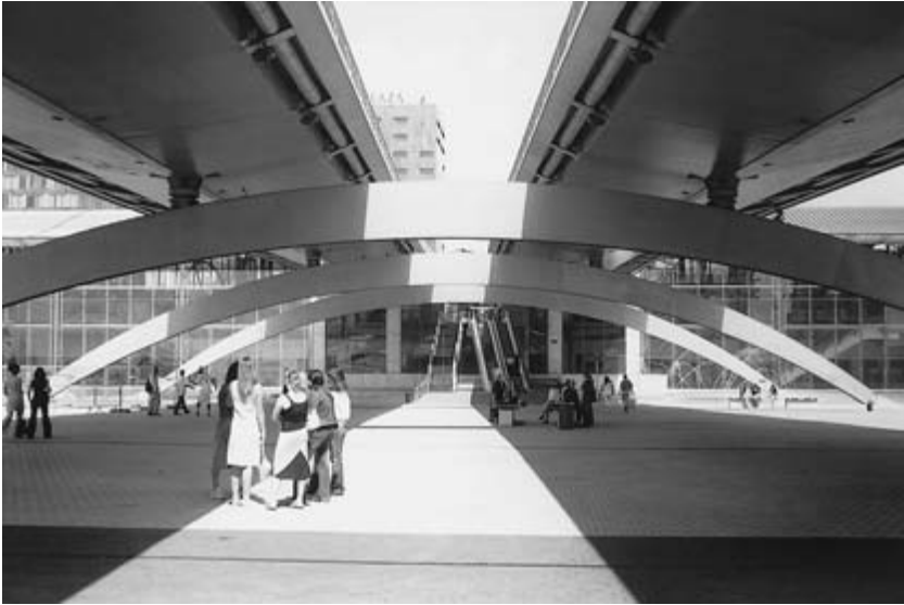
Fig. 17.4 Concrete arches supporting elevated roadway, Lille, France.
