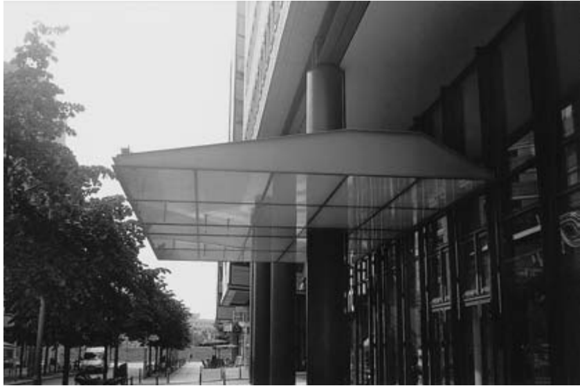
Fig. 23.2 Building with cantilevered canopy, Berlin (detail).
