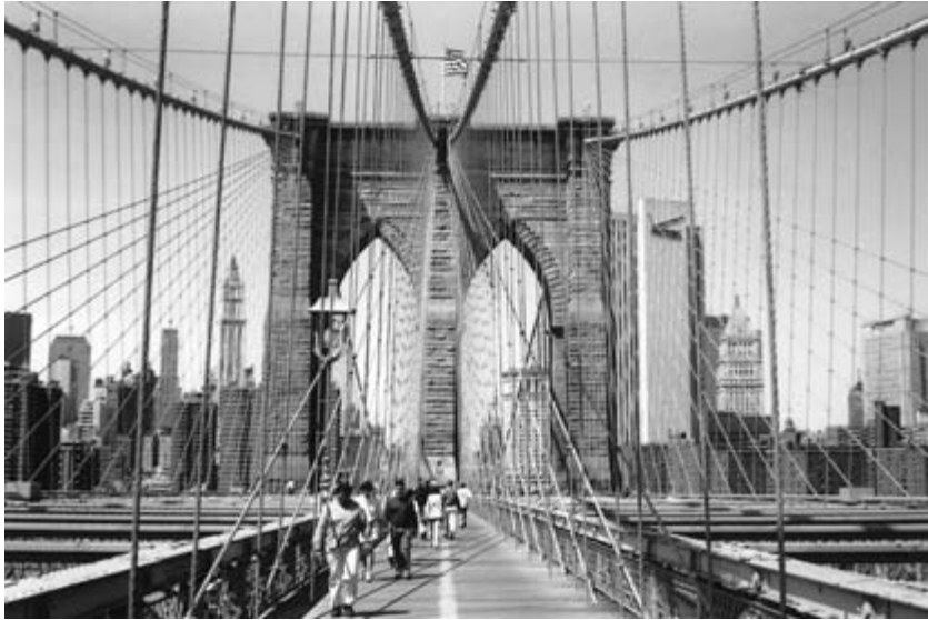
Fig. 3.15 Brooklyn Bridge, New York City.
