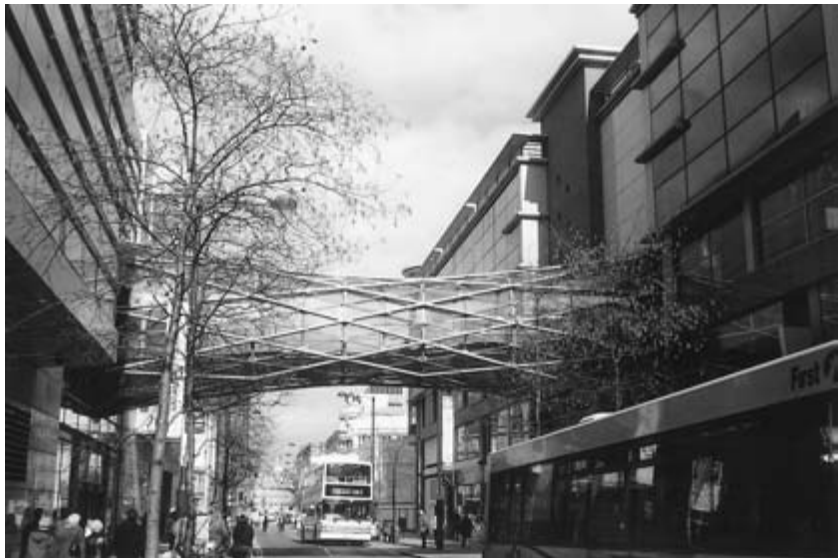
Fig. 21.2 Steel footbridge, Manchester.
