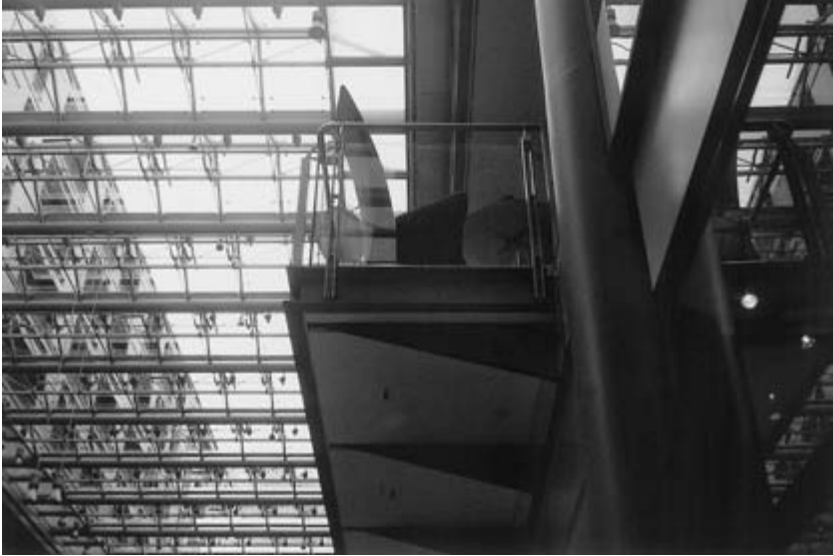
Fig. 16.25 Cantilevered balcony in shopping centre.
