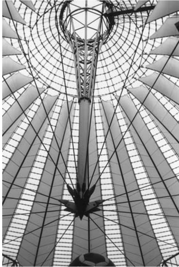
Fig. 17.1 Roof of Sony Centre, Berlin.
